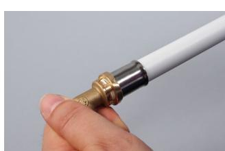
Lubricate the pipe internal surface with lubricants suitable for the system materials and use.
